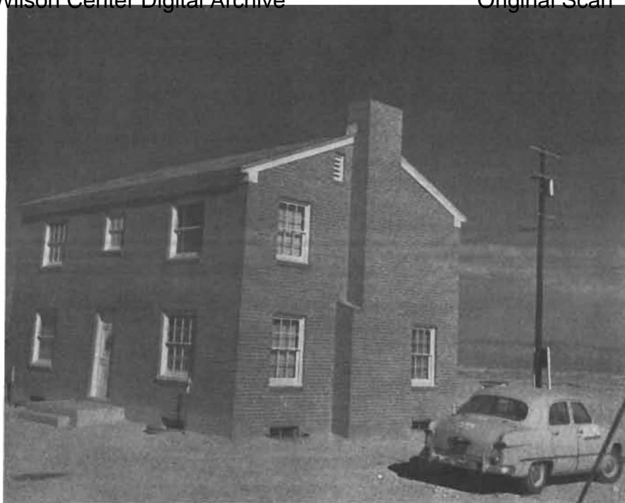
Plate 2 House at 1 mile from ground zero — Before
